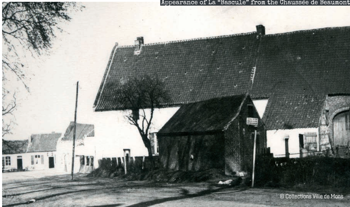
Appearance of La "Bascule" from the Chaussée de Beaumont.
